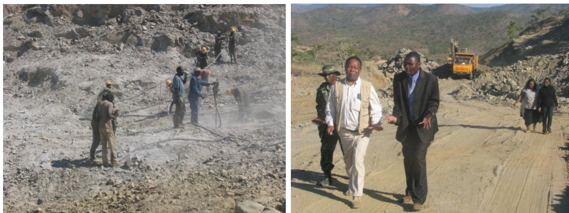
The Karonga-Chitipa Road under construction
