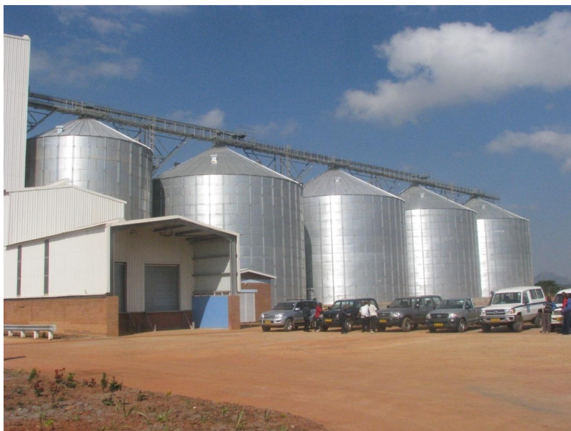
Grain silos constructed as part of National Food Security strategy
