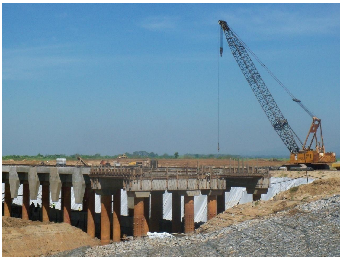
Work in progress on the Nsanje World Inland Port
