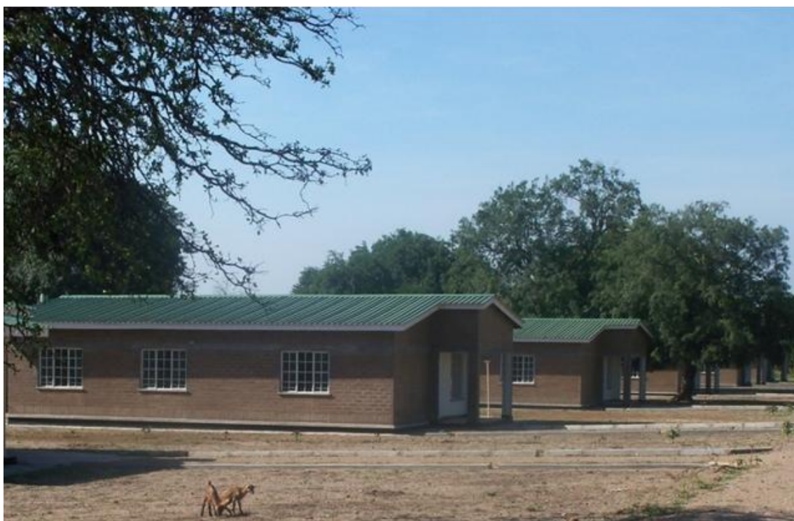
Ministry of Health staff houses at Ngabu in Chikhwawa constructed under the Umoyo Staff Housing Project
